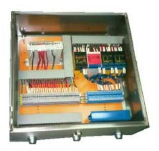
This enclosure is rated NEMA 4X or 12 and contains the additional interface between the machine mounted electricals and the customer's DCS, which controls the centrifuge operation. Specifically, it houses the necessary components such as vibration monitor, speed monitor and intrinsically safe barriers for Class II, Div. 2 systems (shown) or Class I, Div. 1 systems,.
